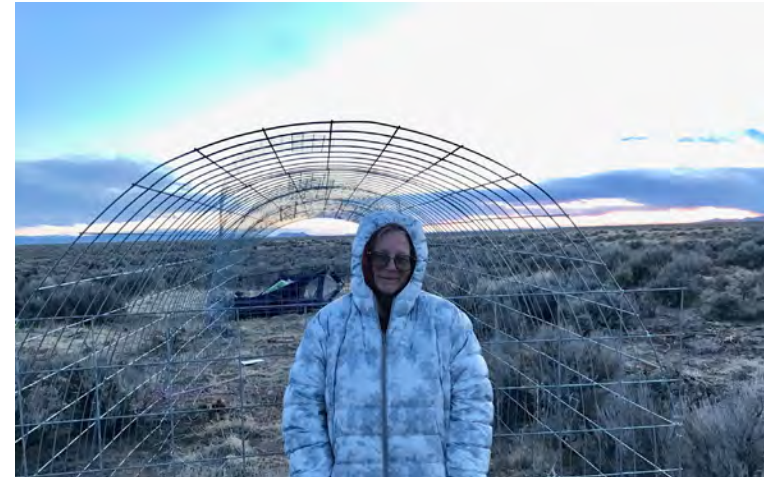
First Day of Desert Fish House Build Welded Steel Livestock Panels, April 2021
